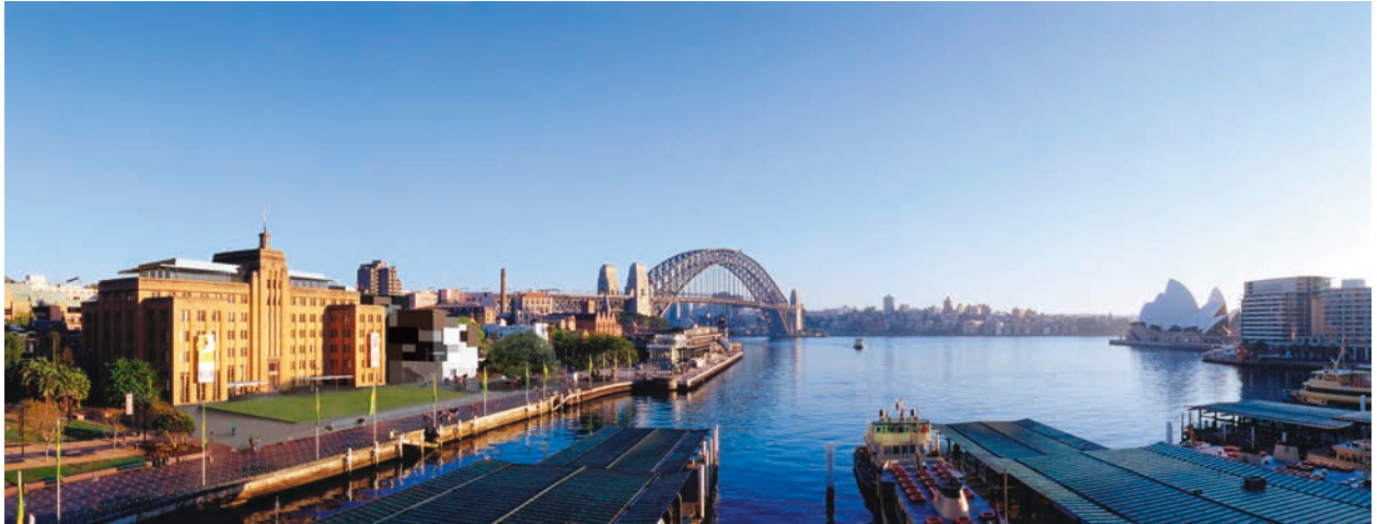
The new MCA as it will appear in March 2012
