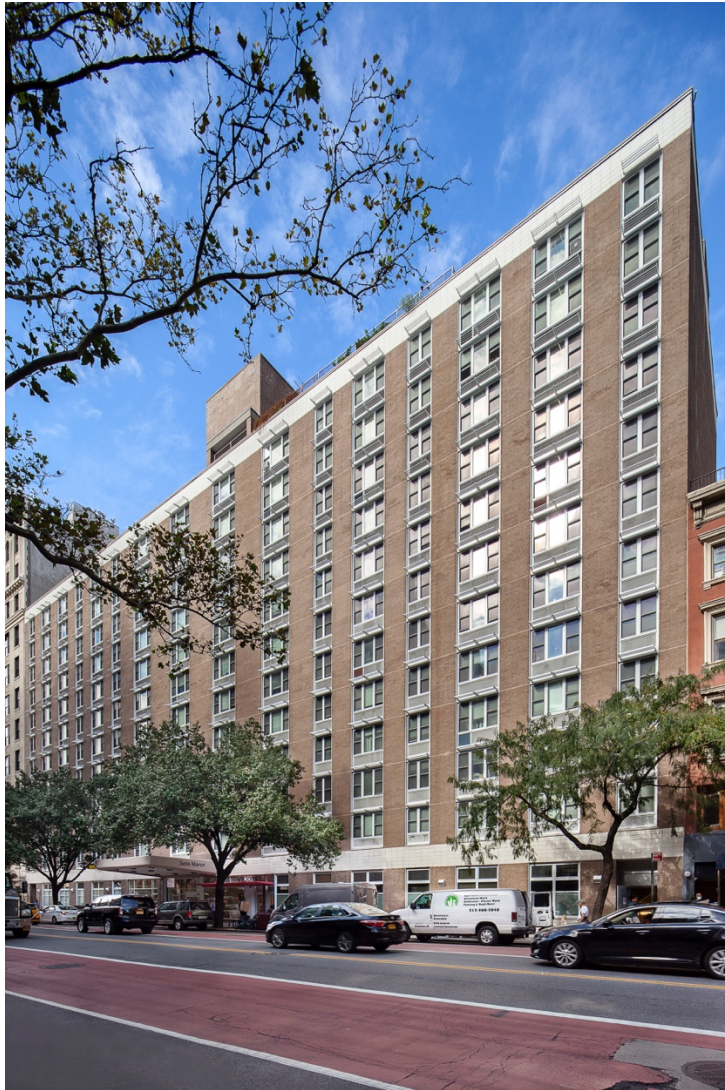
Photo courtesy Magnusson Architecture and Planning.
