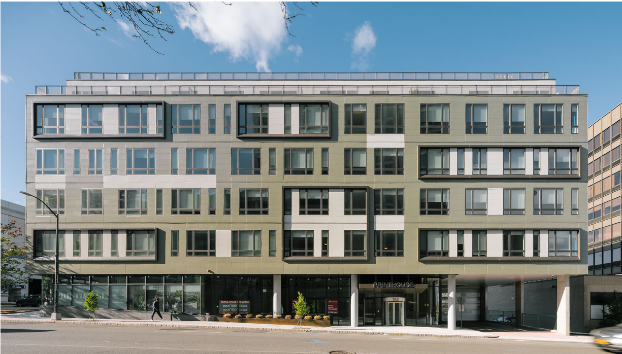
Photo courtesy Magnusson Architecture and Planning.
